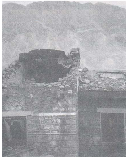
Damaged Building after Pak Shelling
