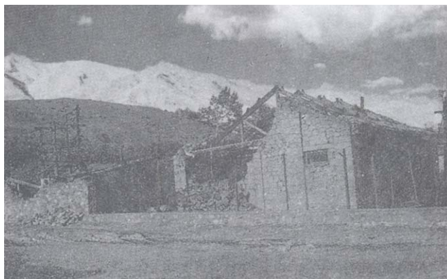
Electric Station at Dras destroyed by Pak Shelling
